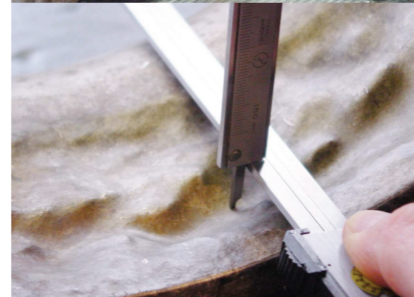
Figure 06: Low temperature corrosion of bottom piece (RTA-type after 28,420 hrs)
